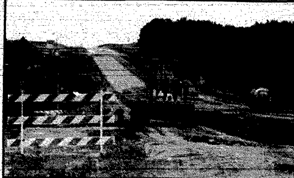
Work continues on the Highway 35 Widening Project including grading on the west end of the project near Pac 'N Save.
